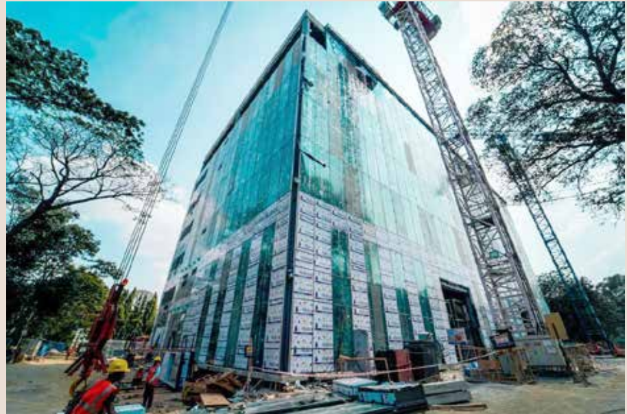
Flight Control System Integration Facility at Aeronautical Development Establishment, Bengaluru
