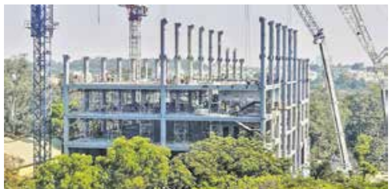
▲ Maiwir Engineering was awarded the fastest structure in India, the 'Flight Control System Integration Facility', at DRDO's Aeronautical Development Establishment, Bengaluru. The seven-storey building was designed using Maiwir Engineering's Composite-Steel Construction Technology.
